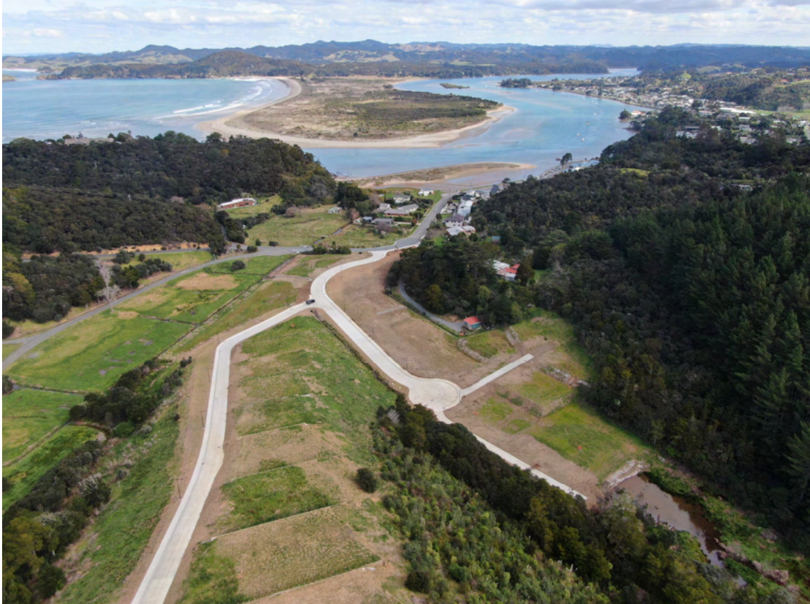
Te Maika Road Core Engineering Solutions Ltd
